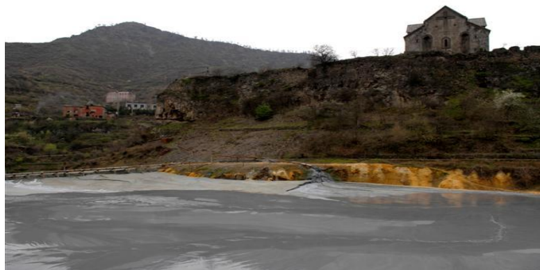
Fig. 7. Tailing dump in Akhtala community is located in close proximity to the church and not far from the school.
